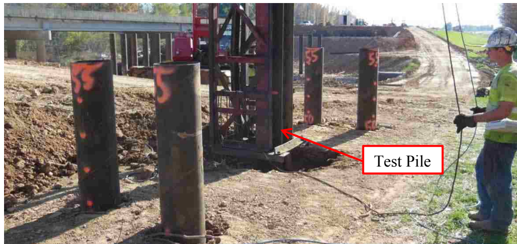
Figure 5.20 A7669 Test Pile Installation
