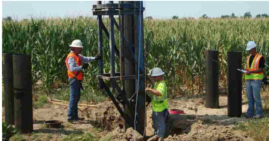
Figure 5.5 A7956 Reaction Pile Installation
